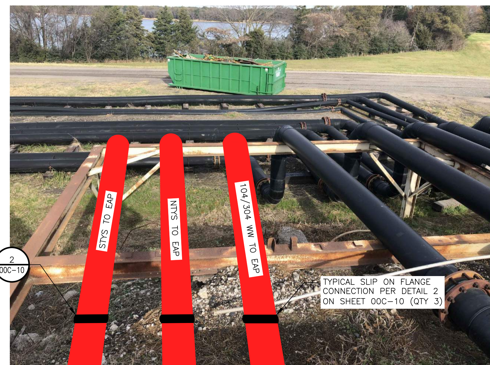
TERMINATION DETAIL C AT EXISTING PIPE RACK (C) NOT TO SCALE 00C-09
